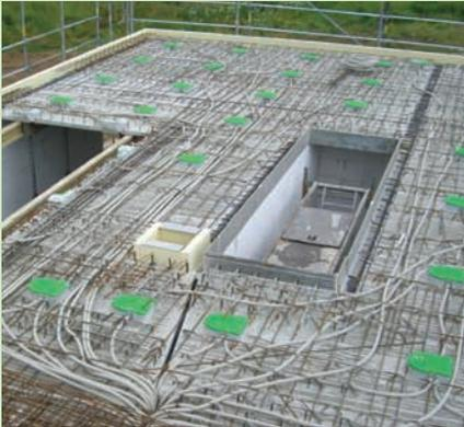
The commonly-used NYM sheathed cables may be installed in concrete, with the exception of concrete which is stamped or vibrated during pouring. According to **VDE 0276**, high-voltage NYY cables may, however, be used without restriction in concrete. However, in comparison with NYM, a considerably larger minimum bending radius must be complied with.
