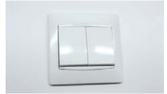
03 Install the cover plate of the switch
