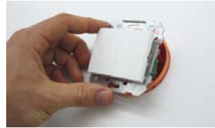
02 Install the switch over the switch coupler
